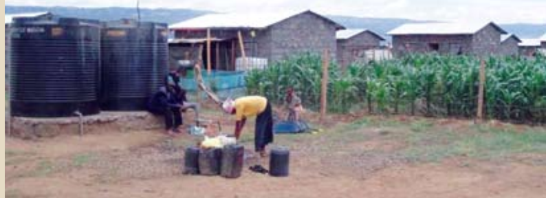
Habitat for Humanity Kenya completed IDP houses in Maai Mahiu
